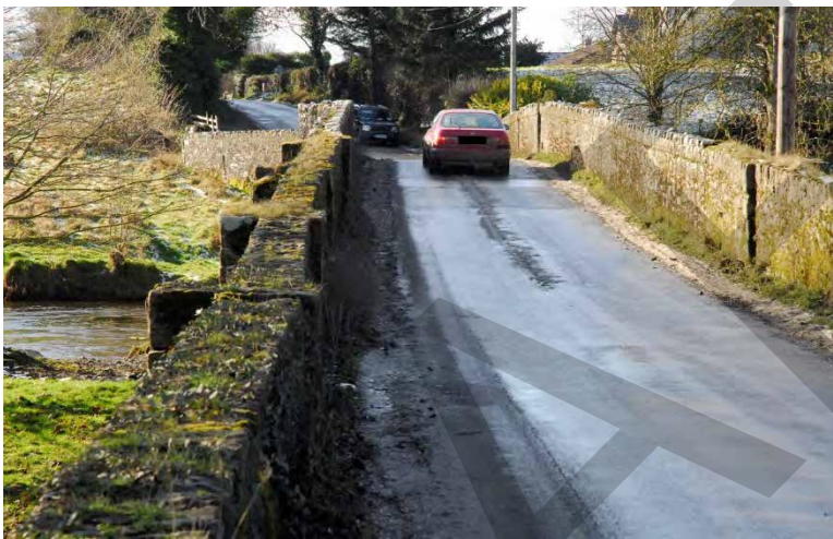
Plate 7. View of car crossing Donaghpatrick Bridge
